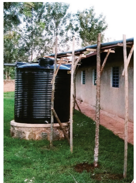
One of the TELD buildings, with a plastic water tank.
